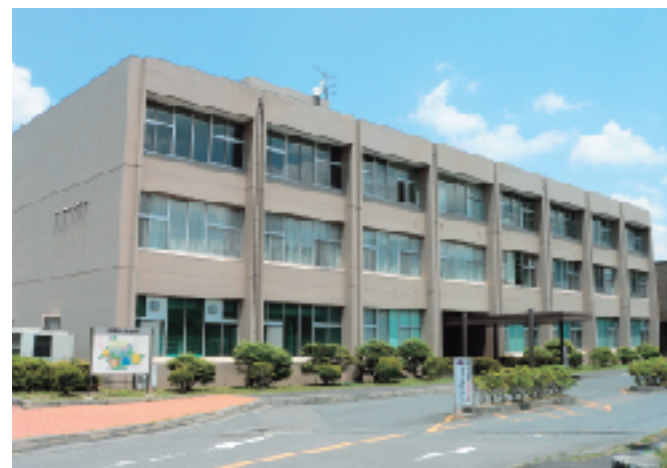
管理棟 Administration Building
